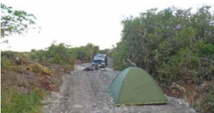
Initial stages of construction of the West Coast Pathway
